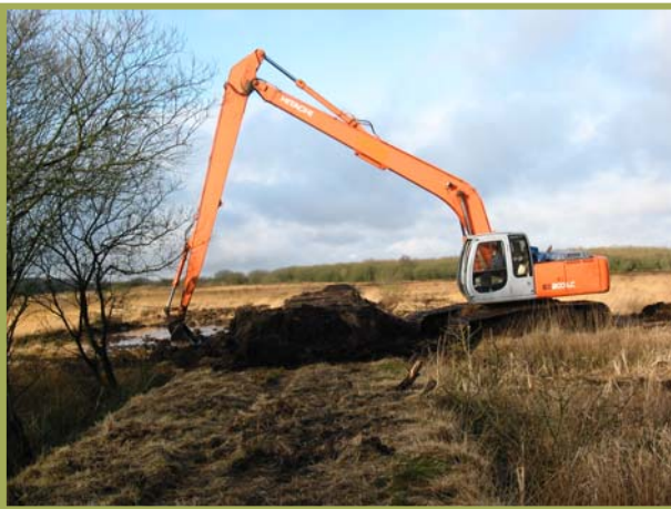
Bund heightening to isolate peat compartments
